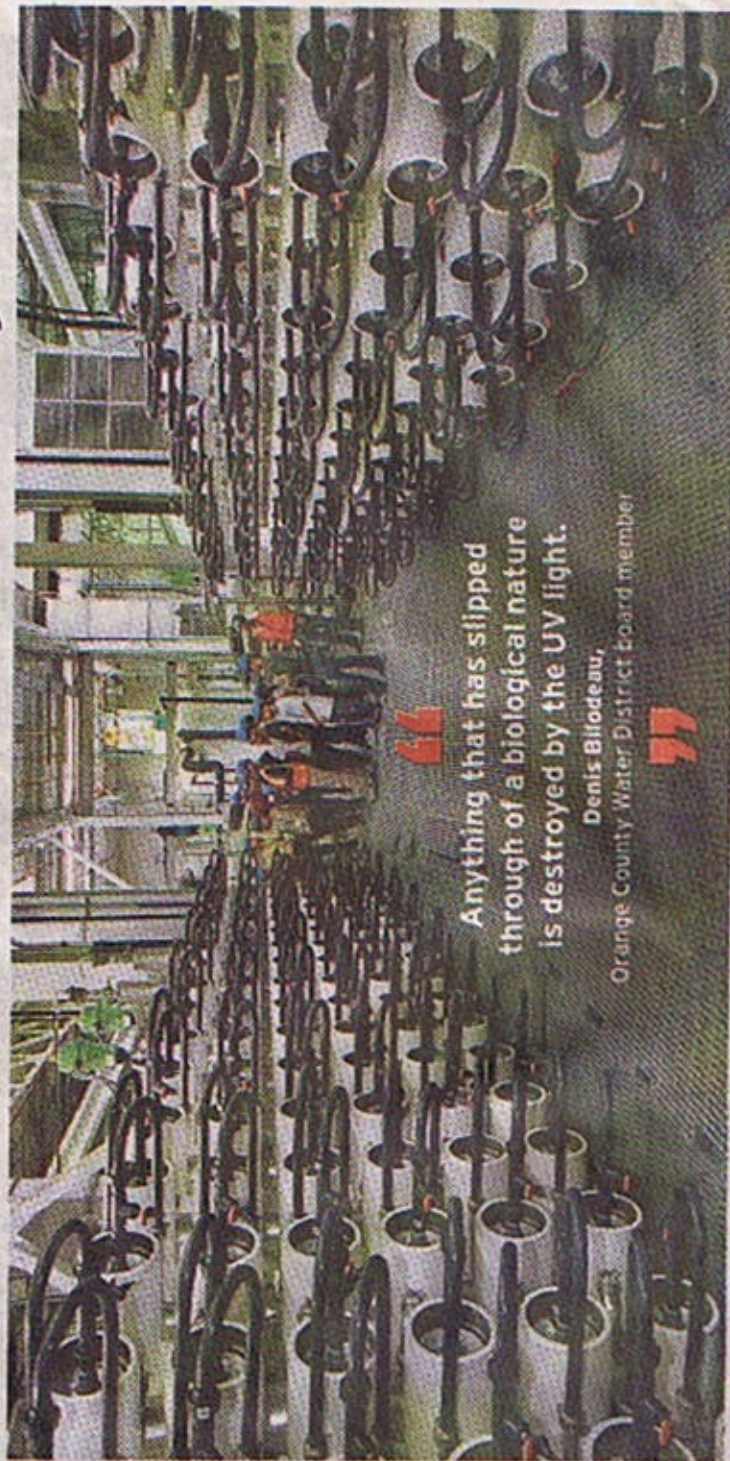
Water is pushed under high pressure through a series of reverse osmosis filters at the Fountain Valley treatment plant. > OC POST
